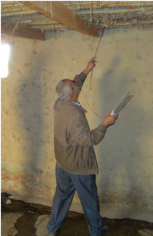
Fig. 34. District entomologist inspecting mosquitoes inside a building in Uzun district, Surchandarya province, Uzbekistan, 2016
