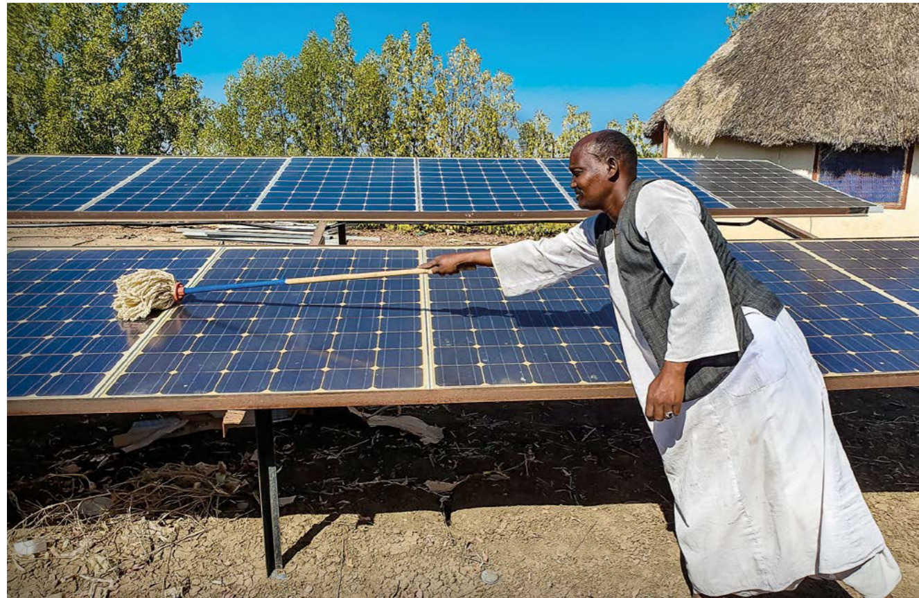
A refugee pump operator cleans the cells that power the solar pump in Um Gargour camp, Sudan.
