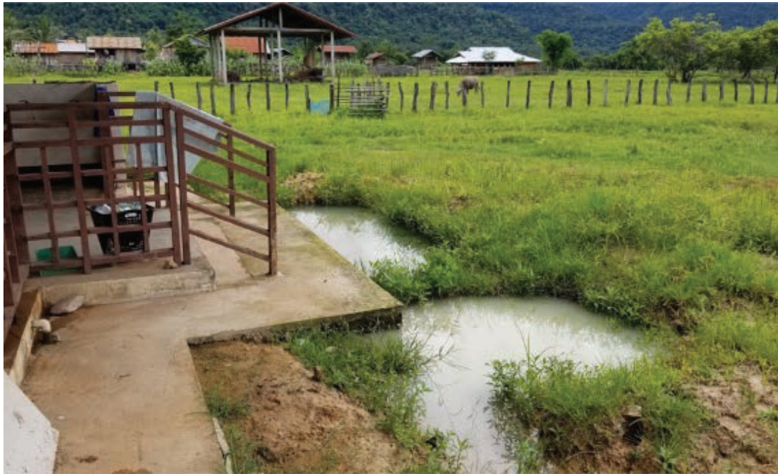
FIG. 30. Flooding due to an extreme weather event
