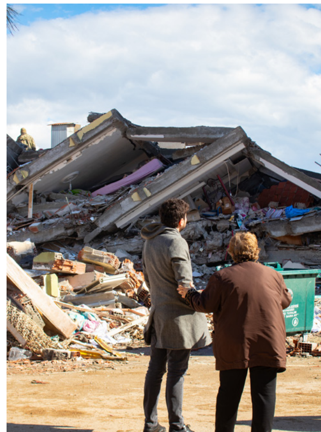
A man and woman look at a collapsed building in Islahya, Türkiye, on 7 February 2023. ©WHO / Ibrahim Al Shikh Ali / Arete
