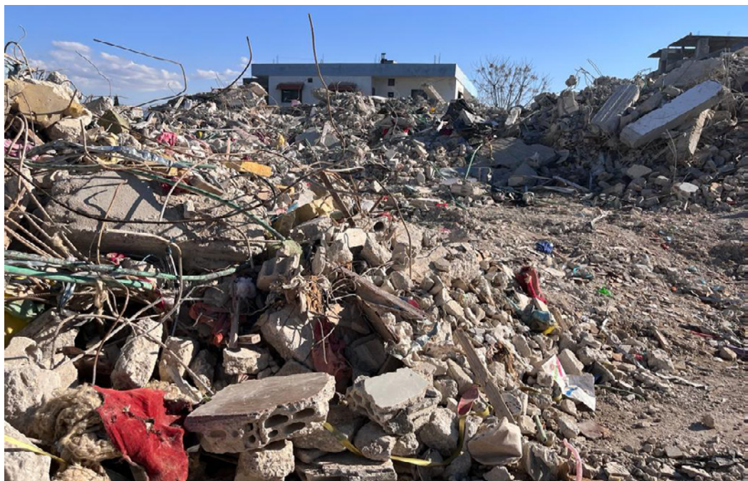
Infrastructure damaged by the earthquake. ©WHO
