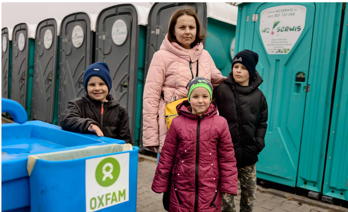
A handwashing point at a registration centre in Przemysł, Poland. Oxfam has started its response in Poland with implementing sanitation like handwashing stations, toilets and showers. "To adapt these facilities to the needs of the refugees we are applying innovative ways of working like installing stand-alone toilets. We have installed showers because people have already been on the move before they come here and need to be able to shower for hygiene reasons but also to relax and find comfort. In this way we also give them back their dignity after the traumatic experiences they have gone through." Angus Mc Bride, Oxfam WASH Coordinator. Photo: Tineke Dhaese/Oxfam
