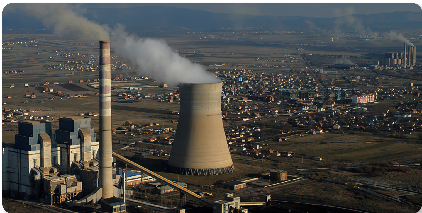
Obilić power plant in Pristina, Kosovo
