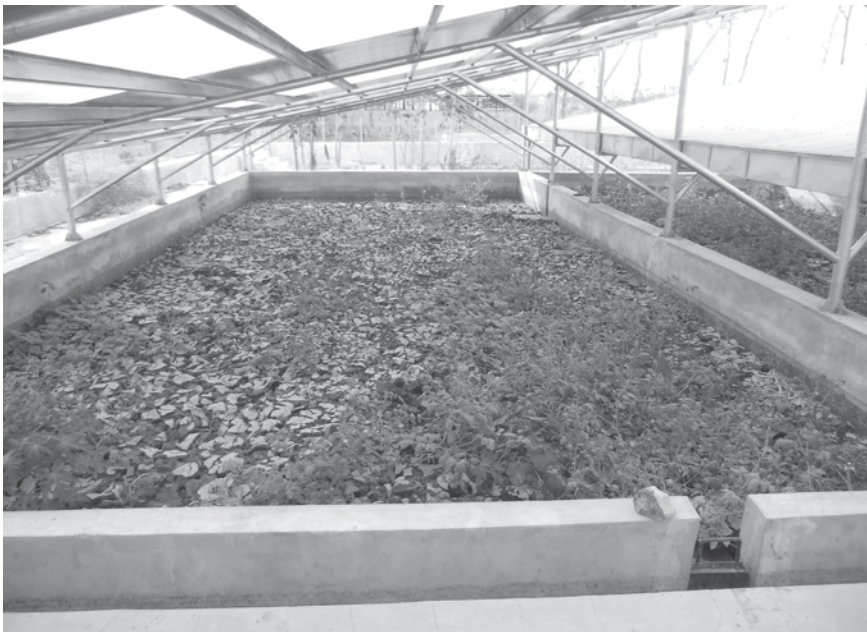
Photo 9.2 Drying bed cover arrangement, Jombang, Indonesia
