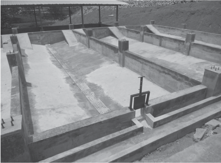
Photo 9.1 Drying beds under construction
