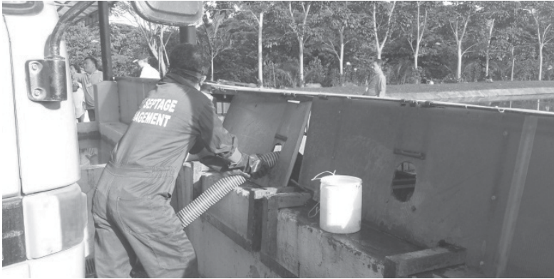
Photo 6.4 Reception arrangement with hinged plastic cover, Dumaguete, Philippines Source: photo by Isabel Blackett
