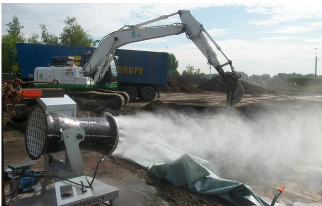
Mitigation measures during site remediation, Buggenhout, Belgium © Public Waste Agency of Flanders
