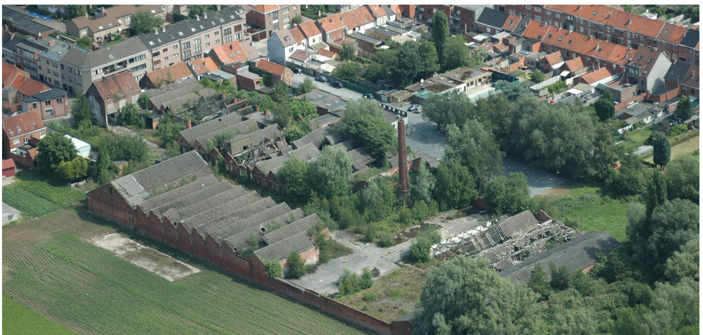
Former textile production plant in Lokeren, Belgium © Public Waste Agency of Flanders
