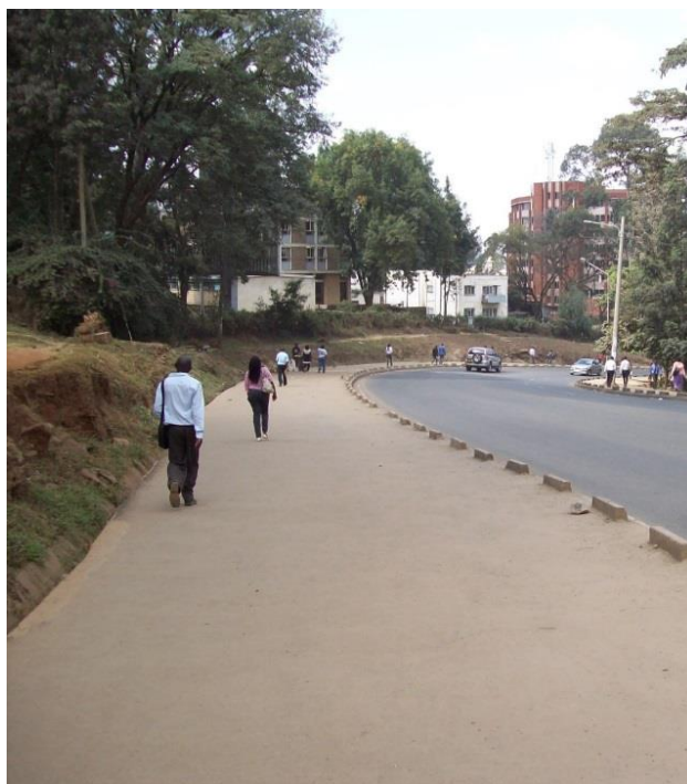
Figure 5: New NMT infrastructure on Haile Selassie Avenue
