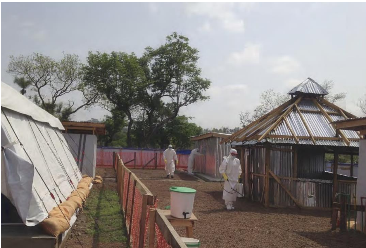
Figure 3 Covered burning pit (at right, pyramid roof), Credit: MDM
