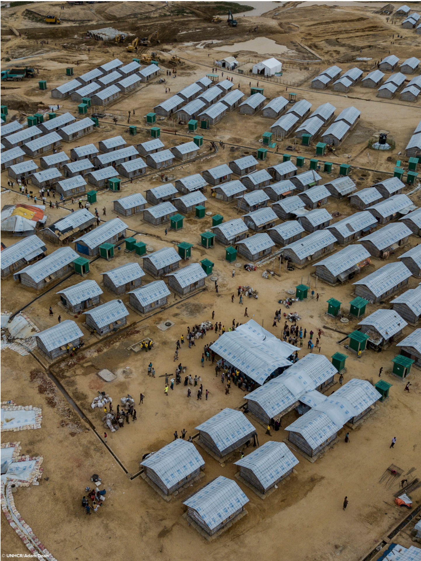
Transitional shelter in Bangladesh
