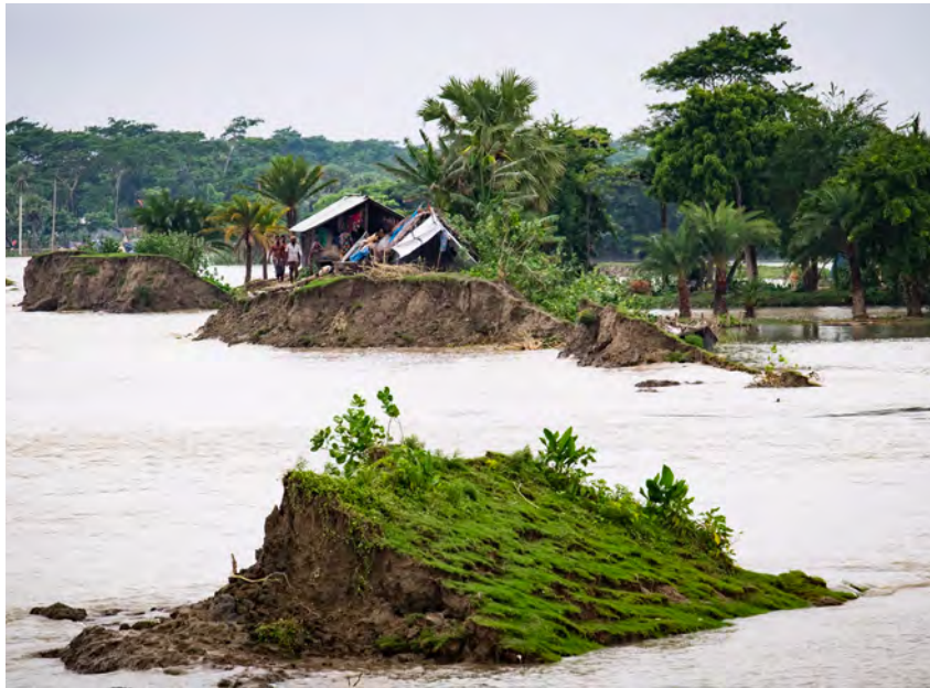
Broken embankments in Bangladesh PHOTO: MAHMUD / MAP / ACTIONAID
