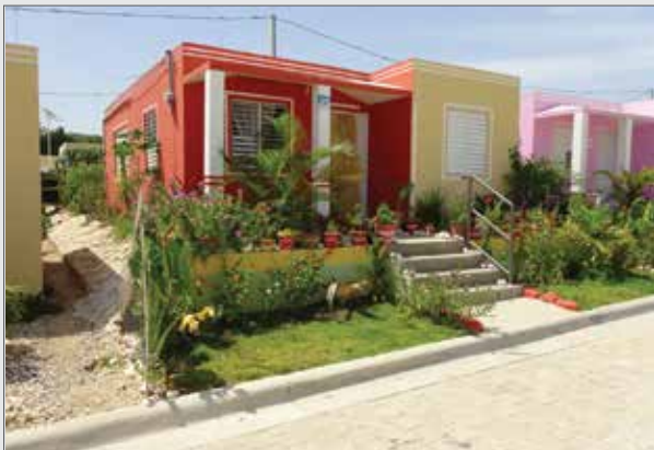
Haut Damier Housing Units
