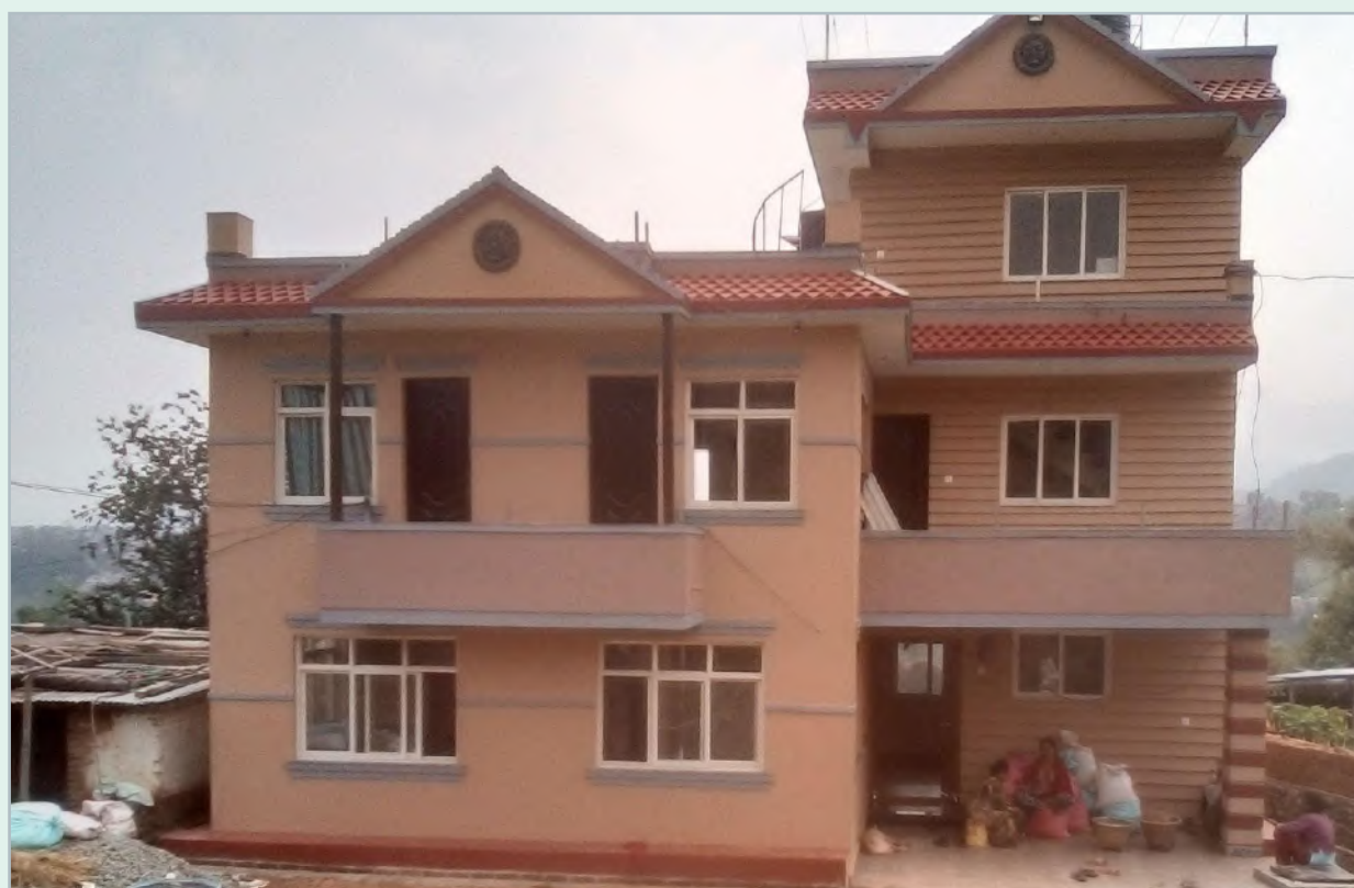
Image 25: Mr. Gurung KC's reconstructed house on Guthi Land Source: HRRP District Team, 2020
