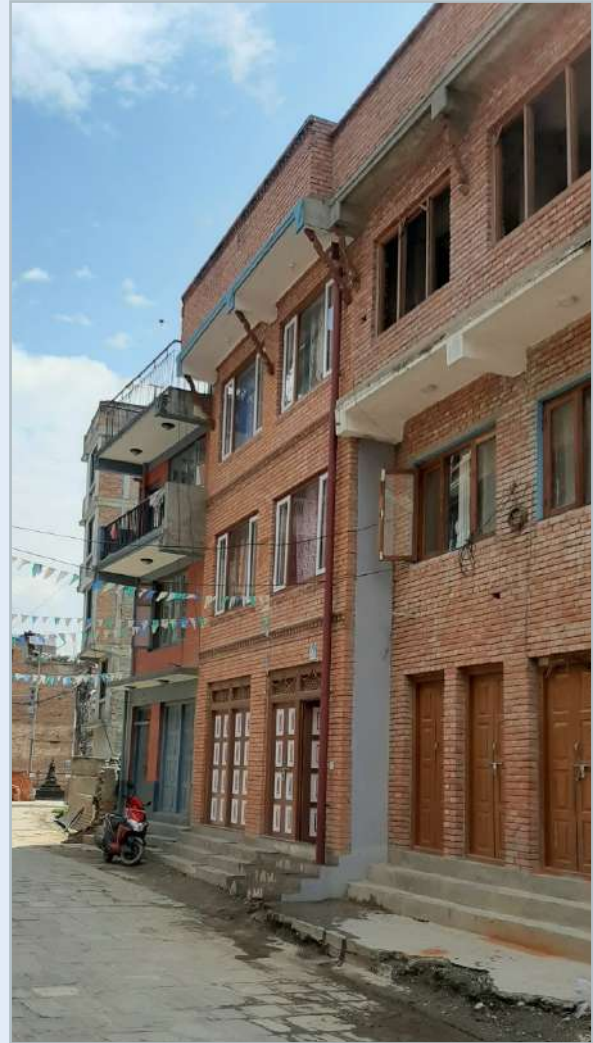
Image 26: Maharjan's reconstructed house (centre) Source: HRRP District Team, 2020
