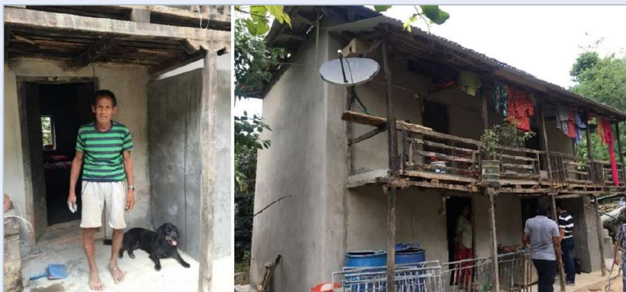
Image 16 (left). Tolak Bahadur in front of his retrofitted house Image 17 (right): Tolak Bahadur's retrofitted house using the Strongback technique, with support from Build Change Source: HRRP District Team, 2019
