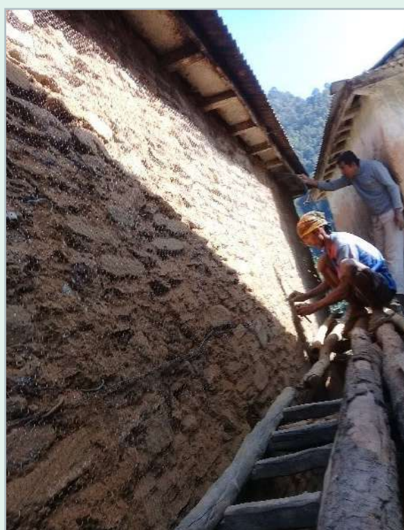
Image 19: Chicken wire mesh “Jacketing” technique being applied. Source: HRRP District Team, 2019
