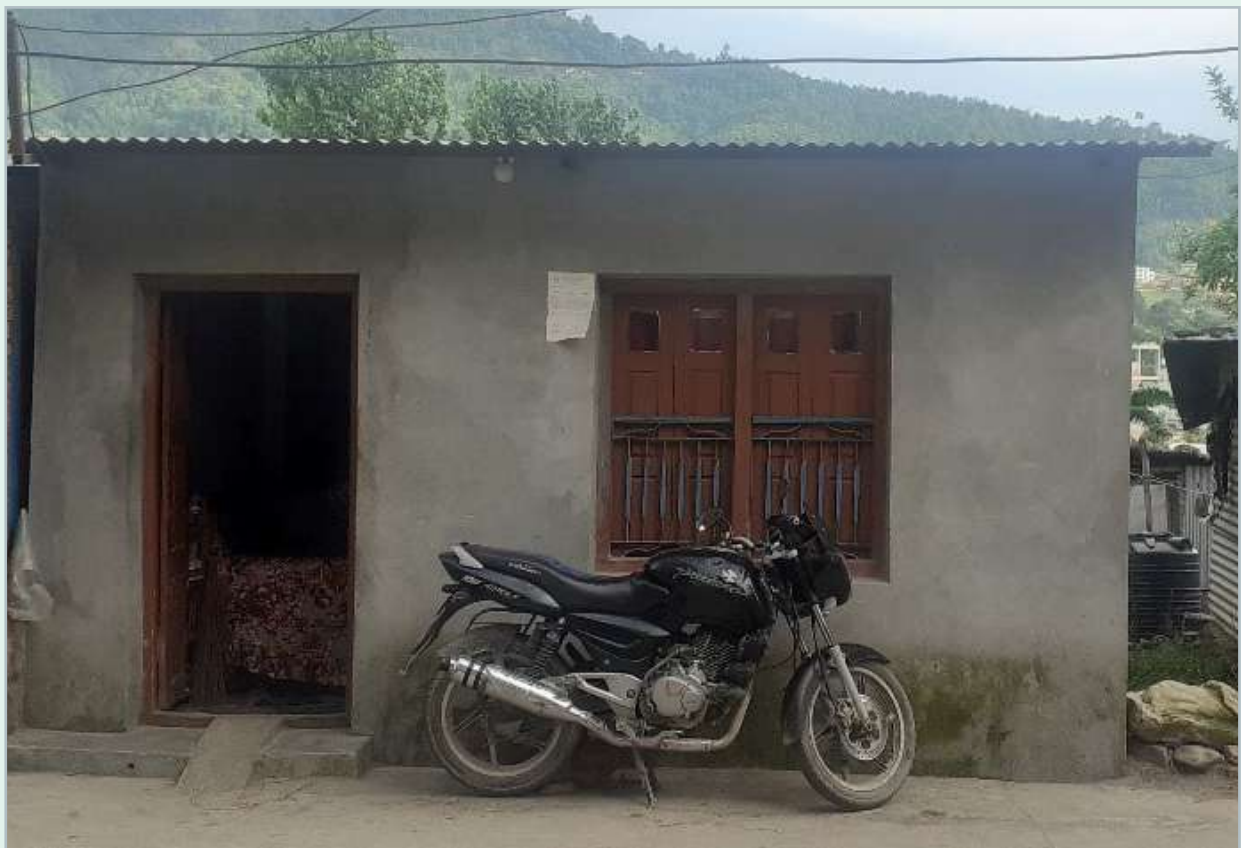
Image 27: Ram Lal Shahi's single storey 4-roomed brick and cement mortar house with a flexible roof Source: HRRP District Team, 2020
