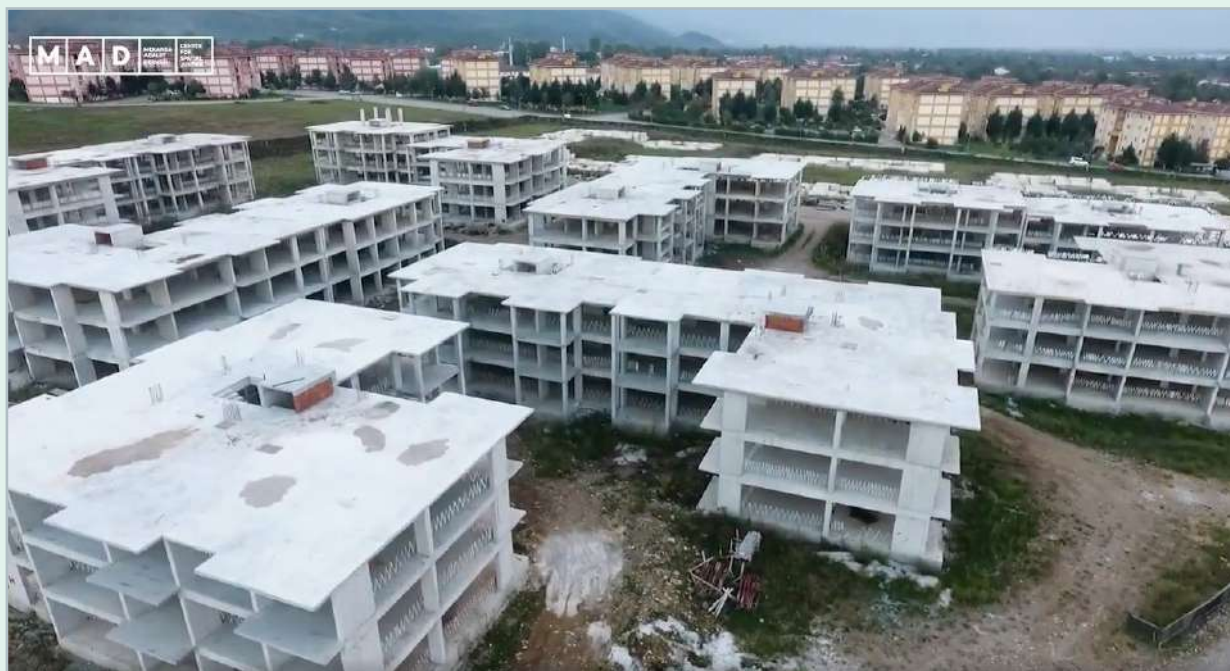
Image 35: Ongoing construction as of late 2019 Source: Mekanda Adalet Derneği
