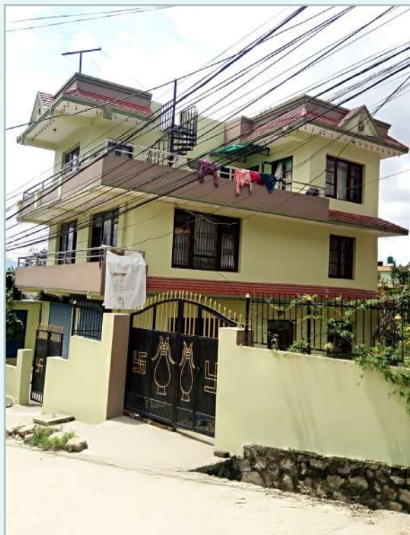
Image 21: Narendra Thapa's retrofitted house. Source: HRRP District Team, 2019
