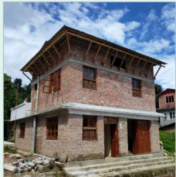
Image 8: Reconstructed house before facade treatment. Source: NSET
