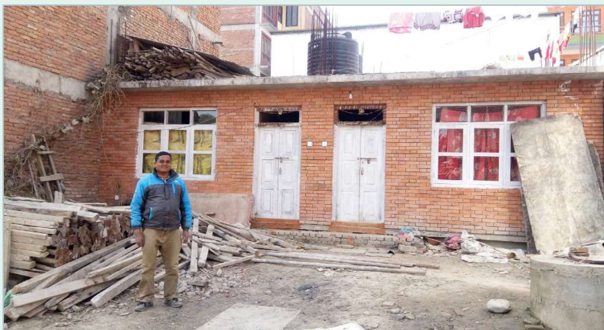
Image 13: Mr. Gosain standing in front of his newly reconstructed house. Source: HRRP District Team, 2019
