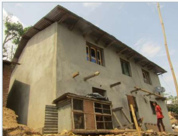
Image 3: Suresh Shrestha's house after being retrofitted. Source: NSET
