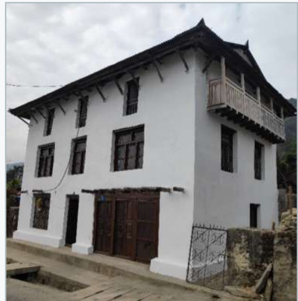
Image 5: Retrofitted house which depicts the culture and architecture of Dwalkha's traditional settlement. Source: NSET
