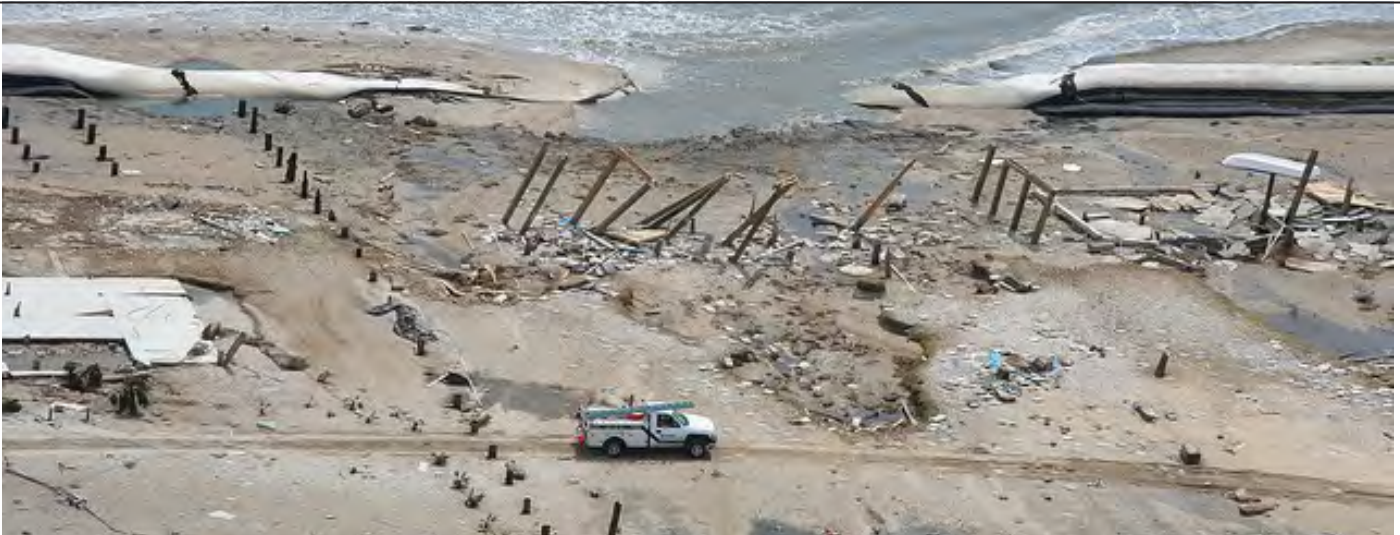
Seawater Inundation Following Hurricane Ike on the Bolivar Peninsula, Texas NOAA, 2008
