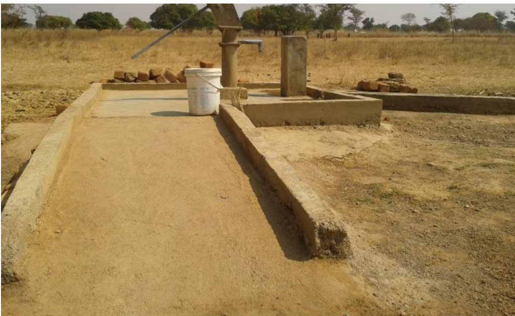
Figure 4.1 A wide ramp at a public water point.
