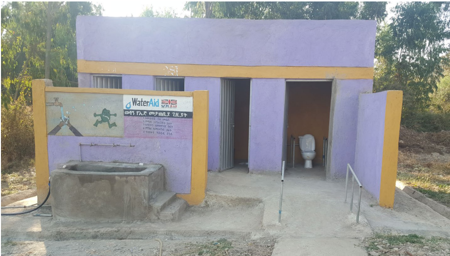
Figure 4.8 Latrine block at a health centre.
