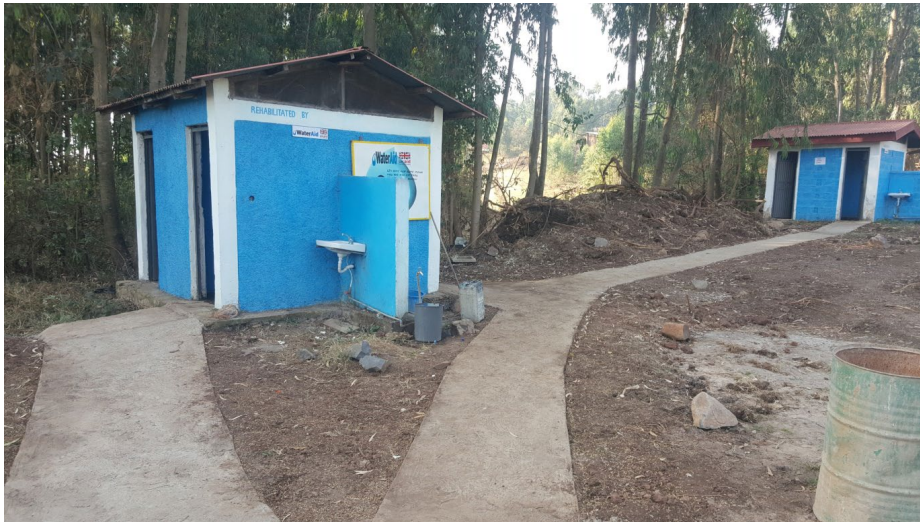
Figure 4.7 Latrine and handwashing facility at a health centre.
