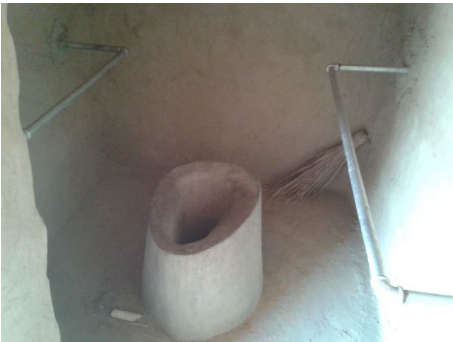
Figure 4.5 An example of a fixed seat with handrails. This would be helpful for many users but there is not enough inside space for a wheelchair user.
