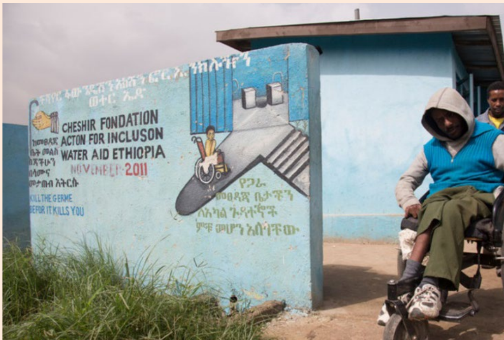
Figure 1.3 Eniyew Yisma outside the school latrine block. Note there are no steps and the entrance is wide so there is plenty of room for his wheelchair.
