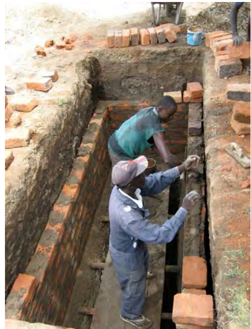
Workers lining a pit with bricks in Kenya.
