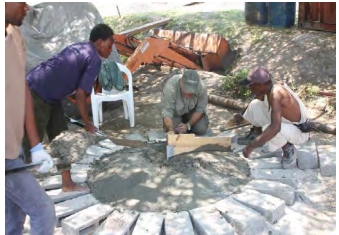
Use the concrete screed to Contour the concrete to the form.
