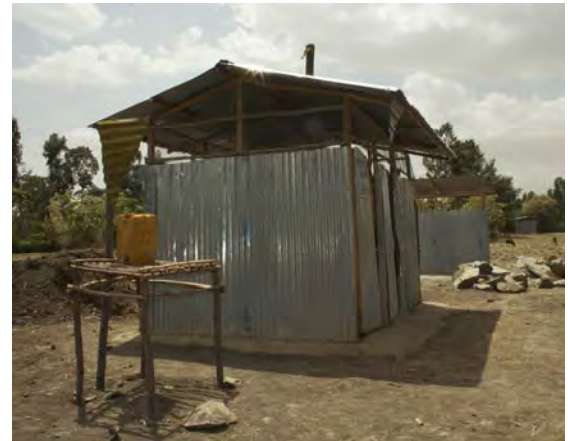
Communal latrine in Ethiopia. The structure is made from corrugated metal.
