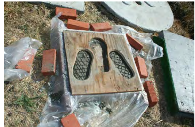
Set the foot pads. Align in front of the key hole.
