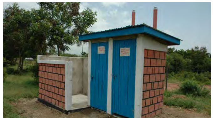
Kenyan latrine constructed with concrete blocks and lined with cement.
