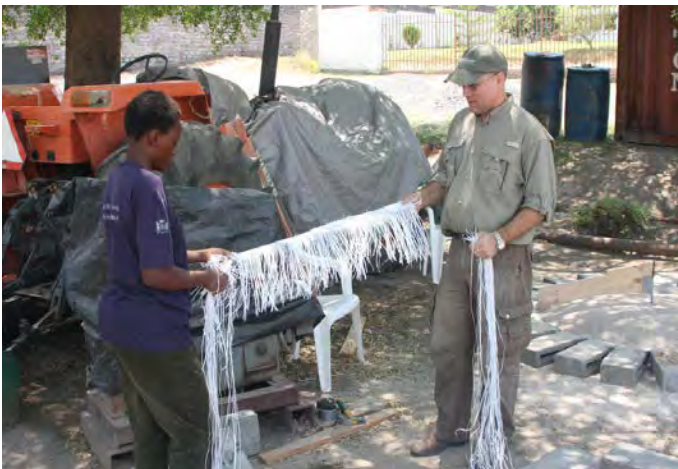
Shredding Fibers for the Dome
