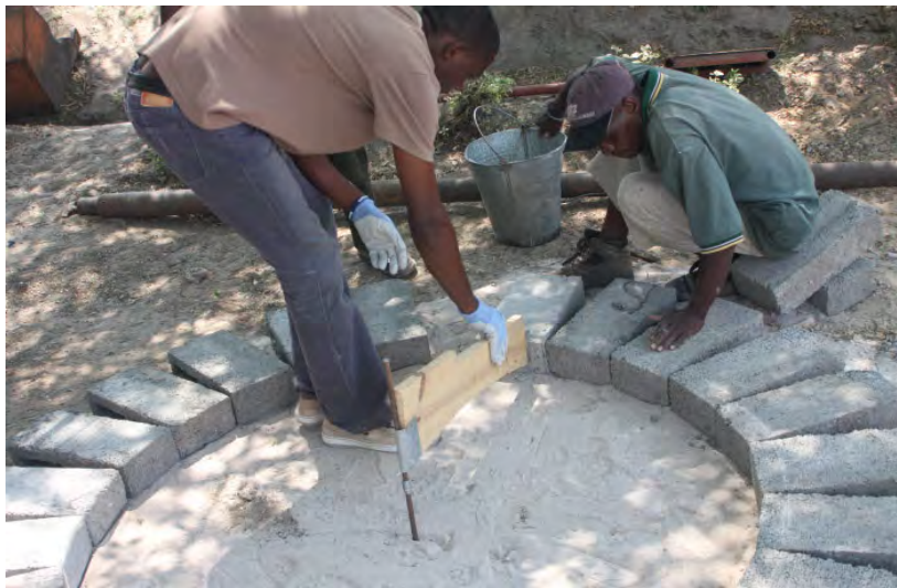
Blocks Create a Frame for the Form
