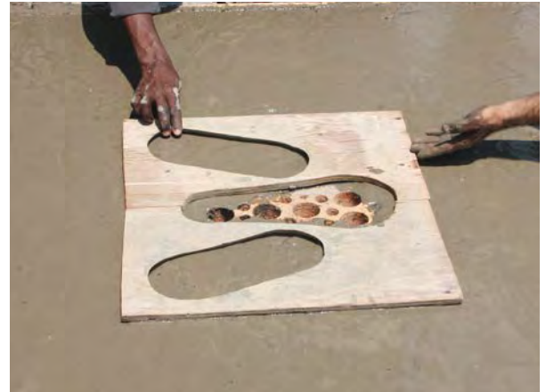
Set the foot pads. Align in front of the key hole.
