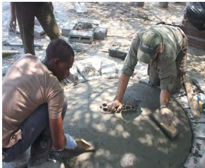
Shine the concrete
