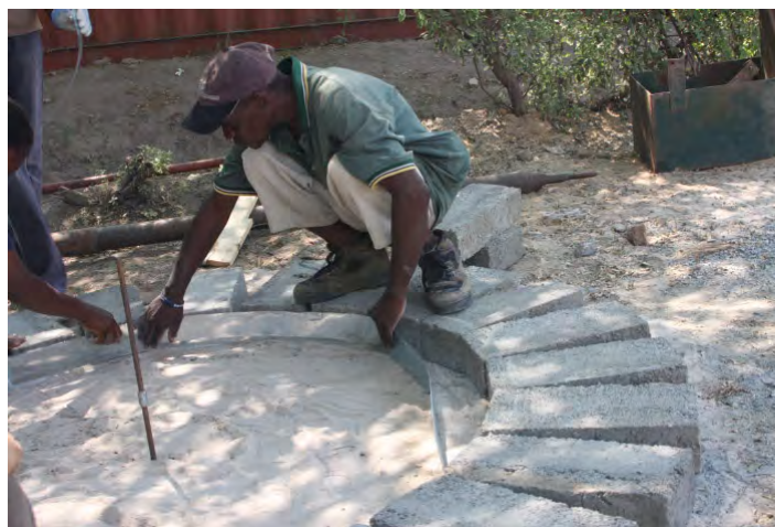
Place Metal Form Inside Brick Frame
