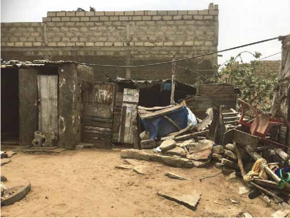
The broken down latrine area of a daara in Dakar, June 23, 2018.
