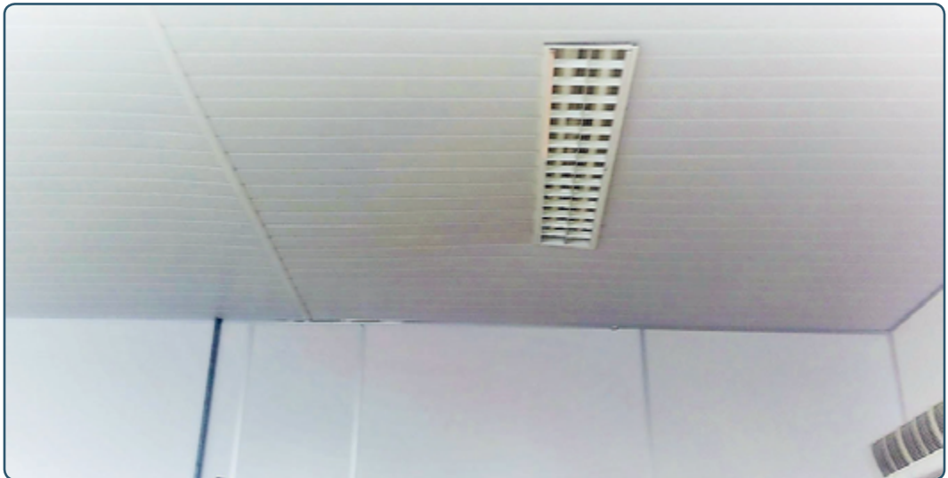
Figure 1. Suspended ceiling
