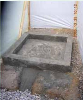
Sanitary pad washing slab inside screened unit
