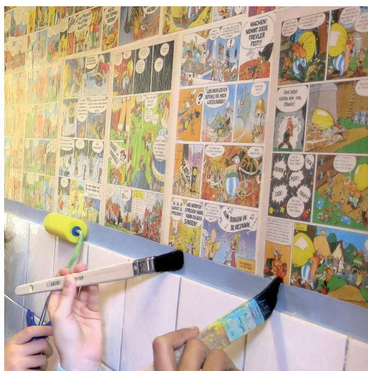
Fig. 7. Pupils implementing the new design of the toilets in the Elisabeth-Seibert-Gesamtschule
