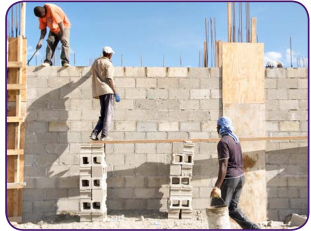
Figure 15: Building the new teaching hospital in Mirebalais, Haiti
