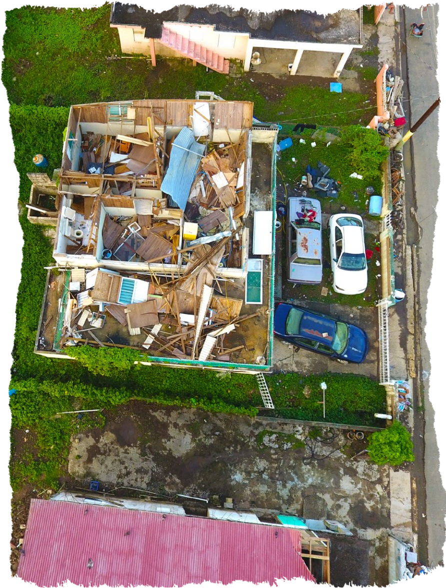
A damaged house in Ingenio, Puerto Rico Source: Dr. Gemma Sou, December 2017
