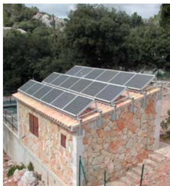
A sewage treatment plant that uses solar power on the island of Majorca in Spain. (Credit: Chixoy)
