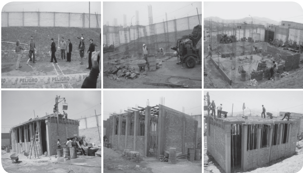
Pilot classroom construction Sept 2012-January 2013 Photographer: Coco Alarcon
