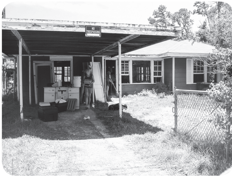
Volunteers repair a house damaged during Hurricane Katrina
