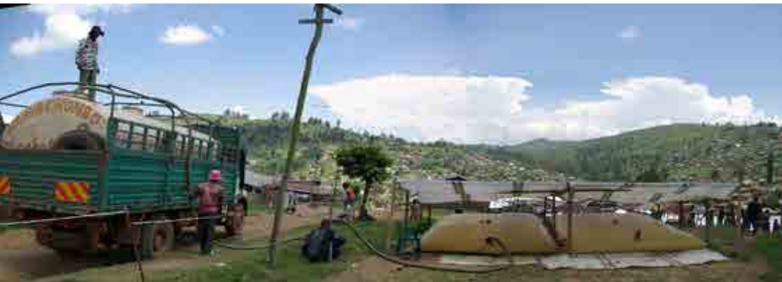
Photo 4: Emptying the tank truck to fill the bladders - North Kivu, DRC © SOLIDARITÉS INTERNATIONALE
