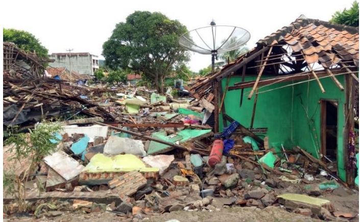
The impact of tsunami/tidal wave in Way Muli, South Lampung. (Photo: PMI)
