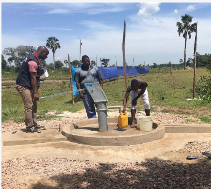
WHO staff using one of the boreholes during one of the monitoring visits in Mwanza.
