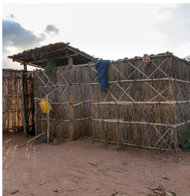
Household latrine made of traditional material, including a handwashing device and a separate area for bathing.
