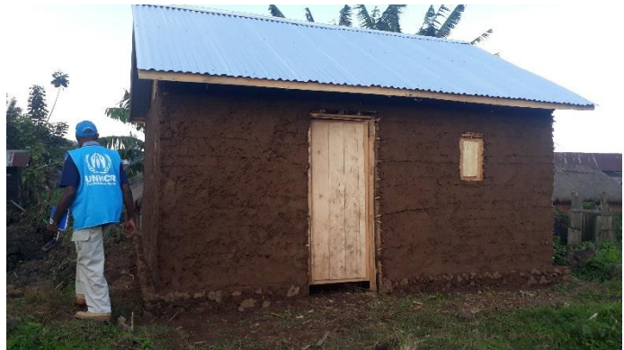
Construction of shelters in Kitshanga, Masisi Territory.
