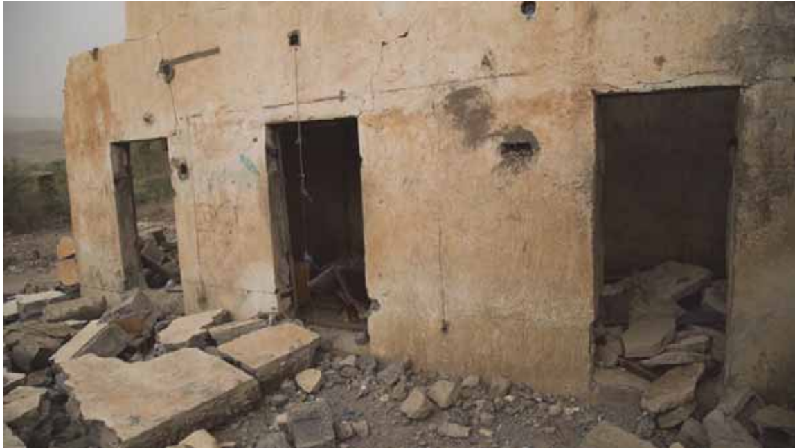
The remains of the home of Omar Ali Farjain, hit by a coalition airstrike on May 12, 2015. Minutes earlier, another bomb struck Abs/Kholan Prison across the street. The two attacks killed at least 25 civilians. Photograph by Ole Solvang. © 2015 Human Rights Watch
