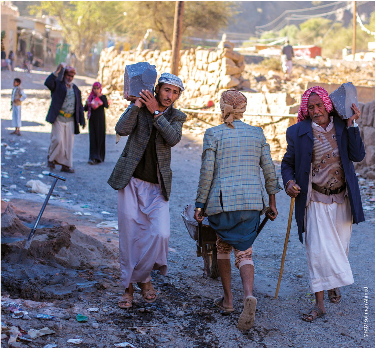
Photo: Villagers help to build a water storage facility in Sana'a.
