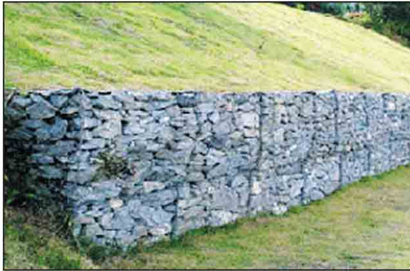
Figure 3-6 Retaining wall built with gabions
