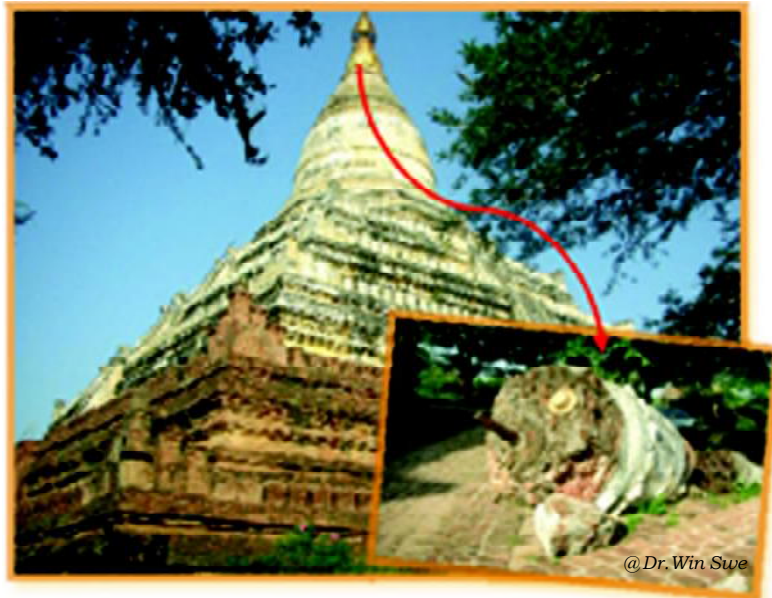
Top of the pagoda shaken down by the 1975 Bagan earthquake, now lying down beside the renovated original pagoda.
