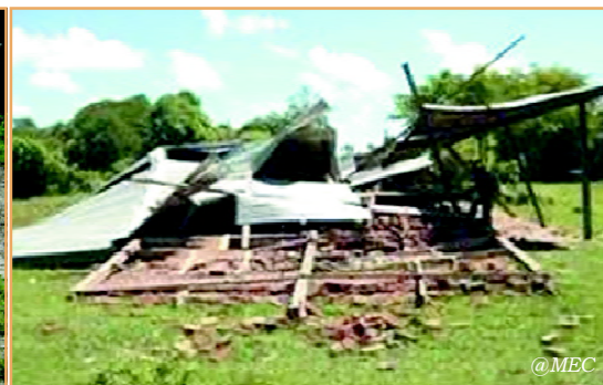
Collapsed primary school during the Taungdwingyi earthquake
