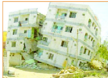
Collapse of buildings during 2001 Bhuj (India) Earthquake
