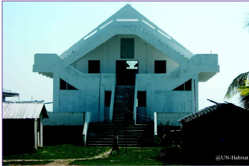
A Cyclone shelter constructed for local community in Tha Gyar Hin Ooe, Kan seik village tract, Dedaye Township
