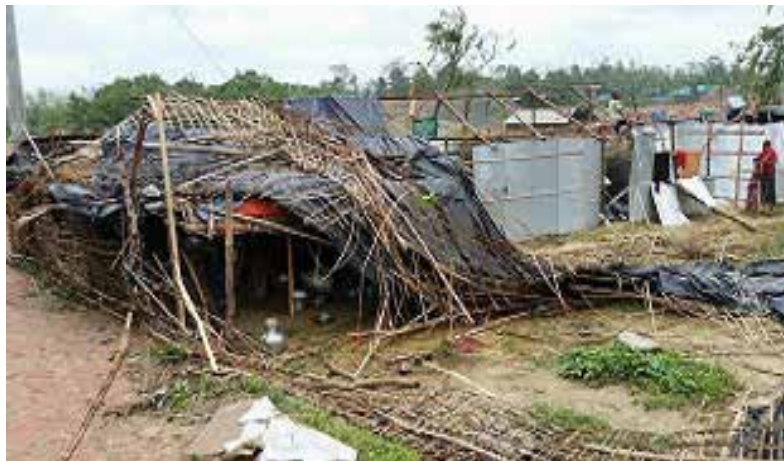
Photo 14: Destruction from Cyclonic Storm Mora
