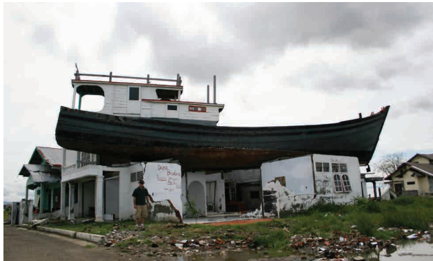
Photo 2: Damage Caused by 2004 Indian Ocean Earthquake and Tsunami
