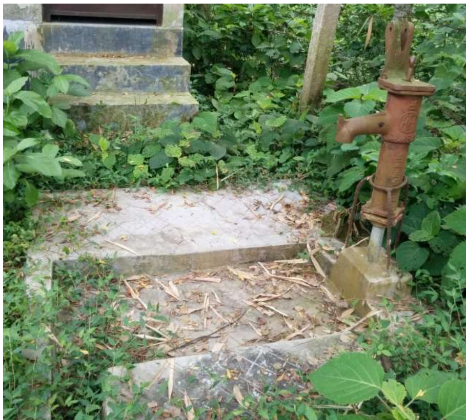
Community Information Centre tube well
