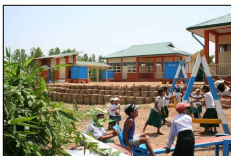
Kungyangone reinforced concrete model school
