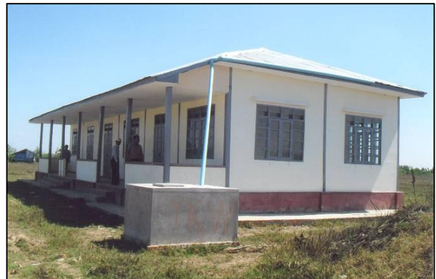
School reconstructed by MoE with rain water storage features
