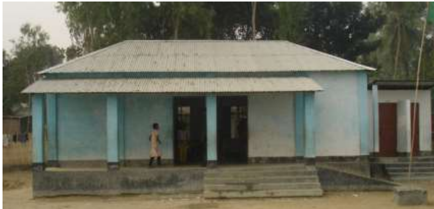
Figure 37: Flood shelter with wheelchair ramp on raised land in Bangladesh. The shelter doubles as a school. Photo: James Pender
