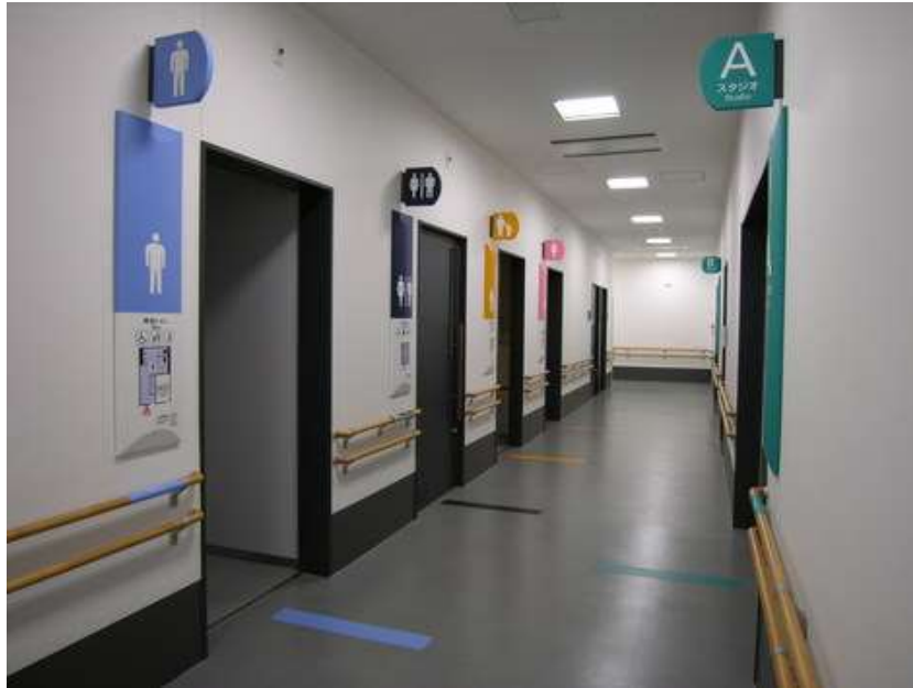
Figure 32: Universally designed corridor, with colour contrasting overhead and wall mounted tactile signage, colour coordinated floor markings. Dual height handrails with Braille information on the top of the handrail. Wide corridors and good illumination. Photo: TOTO Universal Design Laboratory, Kanagawa.
