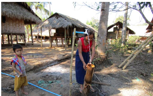
Installing water system to communities
