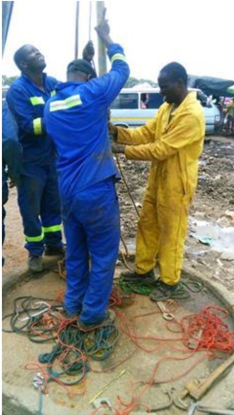
Repairing a water borehole in Harare (Alert 136 Zimbabwe Typhoid). Credit: Welthungerhilfe.
