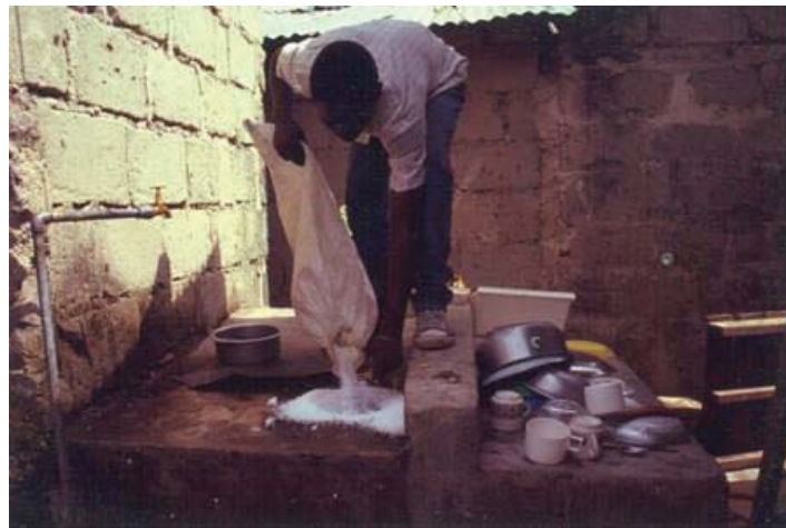
Fig. 21. Treatment of latrines with expanded polystyrene beads (photo courtesy of J. Ensink)
