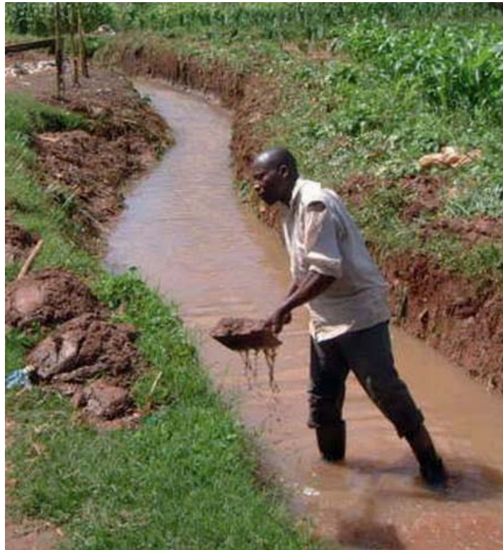
Fig. 26 Environmental management by clearing drains to reduce breeding sites (photo courtesy of S. Lindsay)
