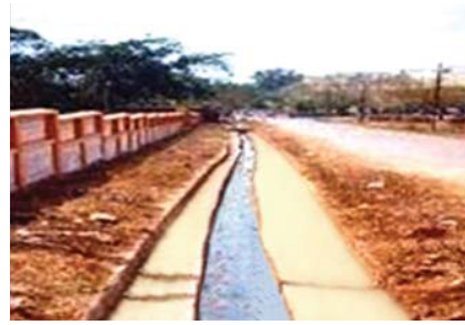
Figure 39. Lined margins of a surface drain ensure free flow of water © Ashwani Kumar
