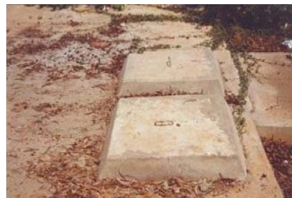
Figure 41. Sealed septic tanks prevent culicine breeding especially of Culex quinquefasciatus © Ashwani Kumar
