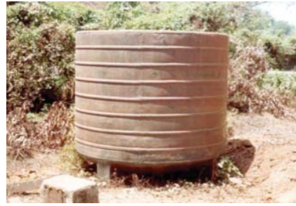
Figure 37. Disconnected overhead tank should be kept inverted © Ashwani Kumar
