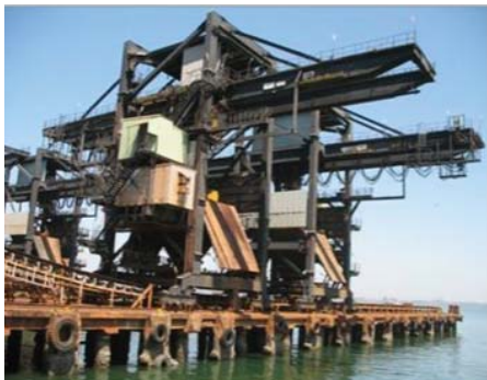
Figure 32. Tyres abutting jetty when filled with rain water can be extremely dangerous in providing the first foothold to any mosquito arriving with a ship © Ashwani Kumar
