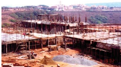
Figure 48. Construction site at PoE with an enormous potential for mosquito breeding © Ashwani Kumar
