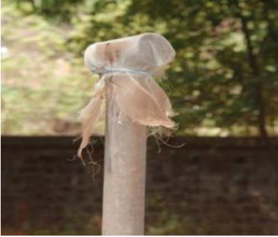
Figure 42. Distal end of vent pipe covered with nylon mesh prevents mosquito entry © Ashwani Kumar
