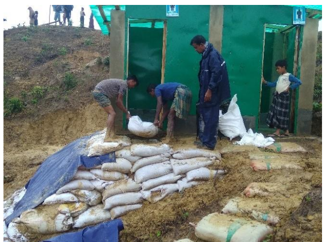
Latrine repairs, Camp 17. Photo Credit: NGO F
