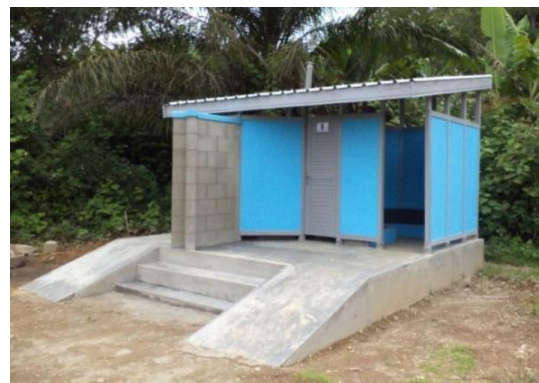
Figure 10: Toilet facility with both step and ramp access (Source: UNICEF)
