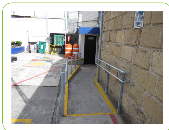
Figure 16: Ramp at school entrance (Source: Janett Jimenez)
