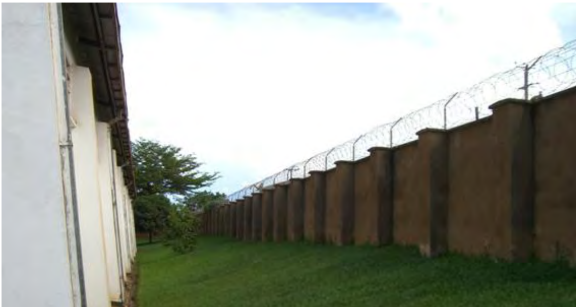
Figure 6.2 Perimeter wall with barbed wire
