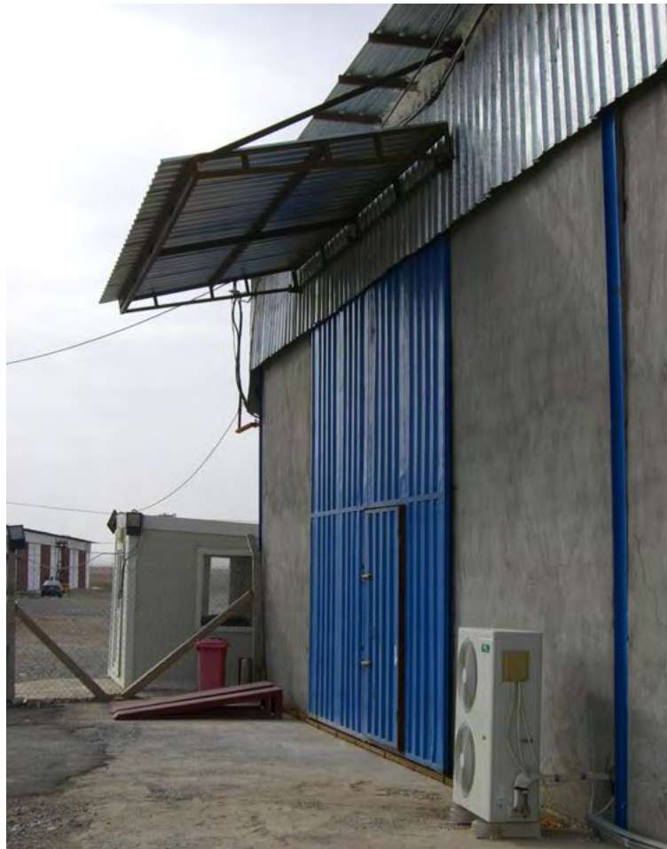
Figure 10.10 Protective roof above warehouse entrance
