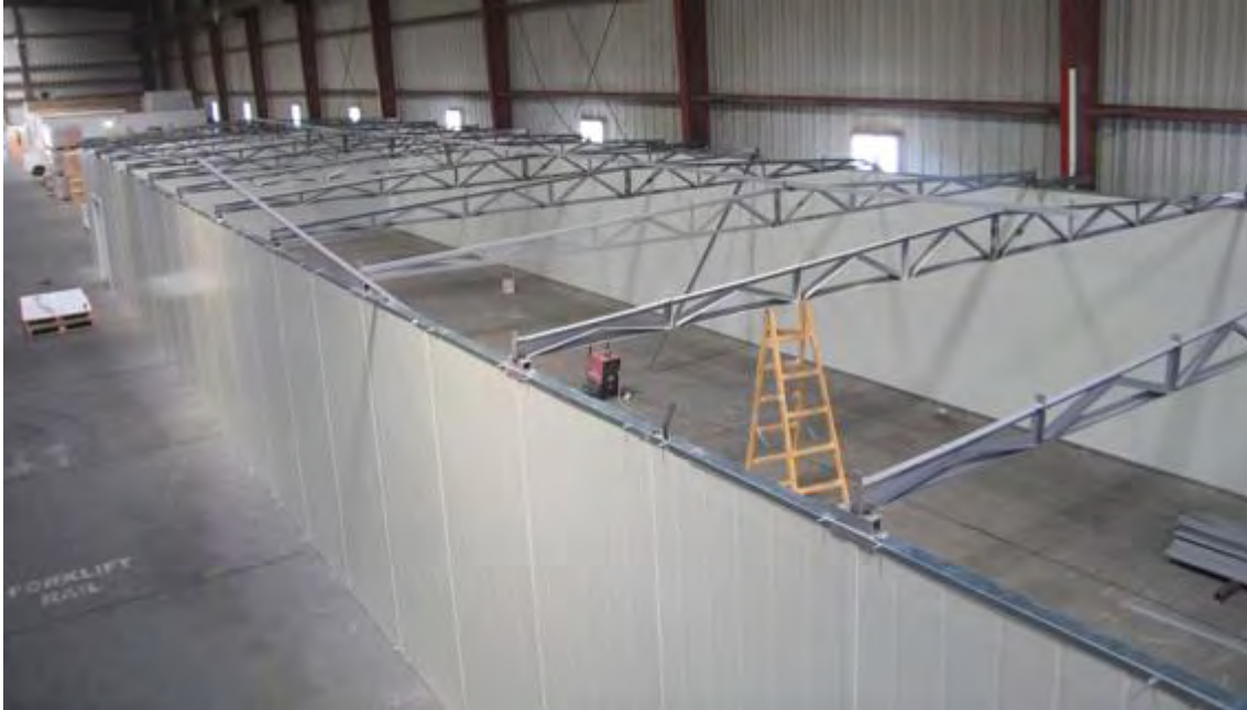
Figure 17.35 Partitioning of store room for cool room
