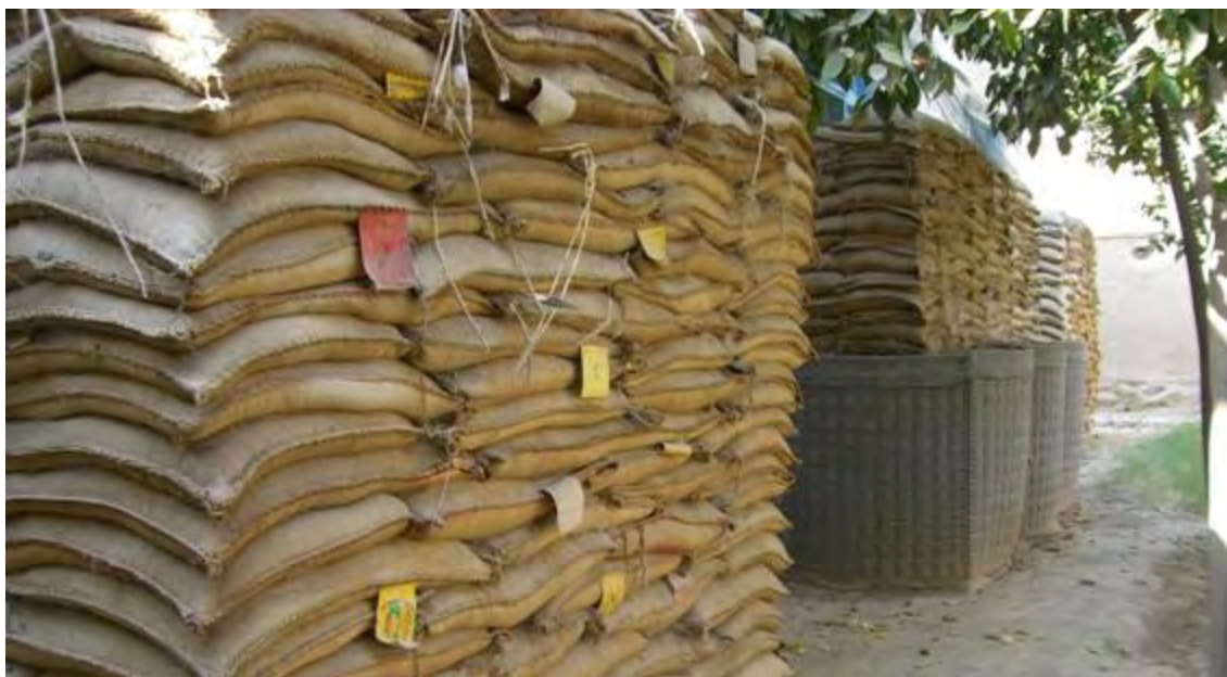
Figure 6.4 Sand bags protecting openings of a building
