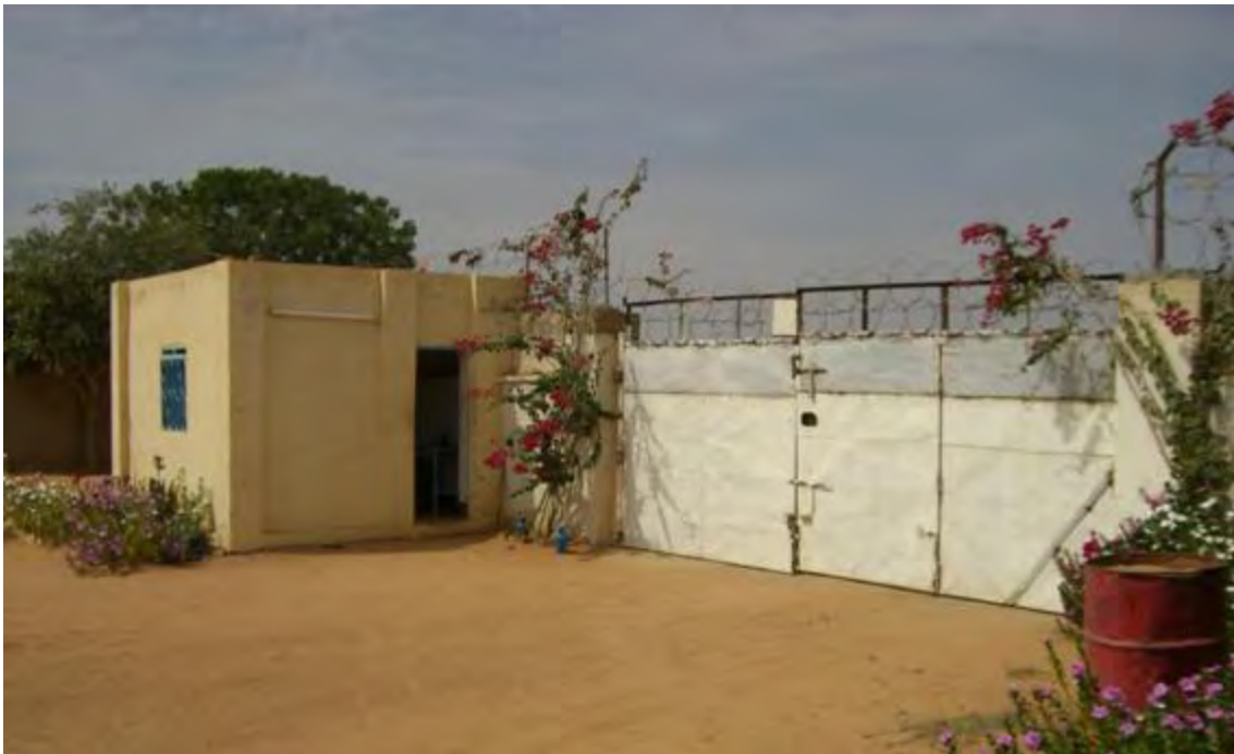
Figure 6.3 Main gate with guard building
