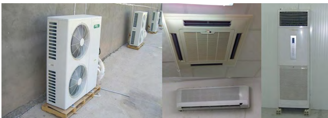
Figure 17.34 Split air-conditioning unit
