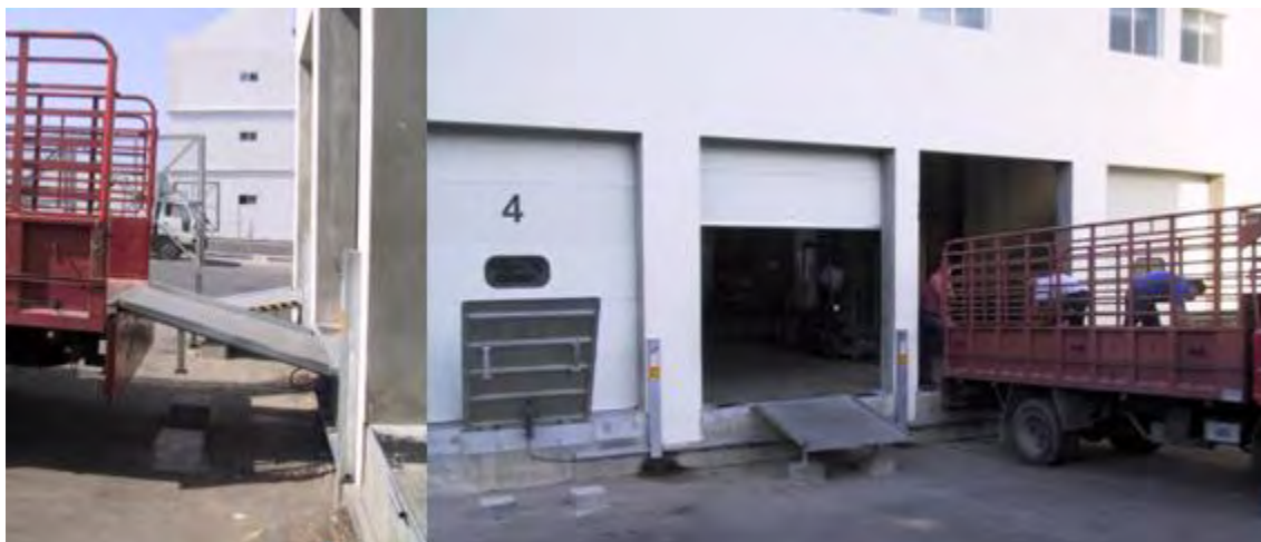
Figure 10.11 Dock leveller
