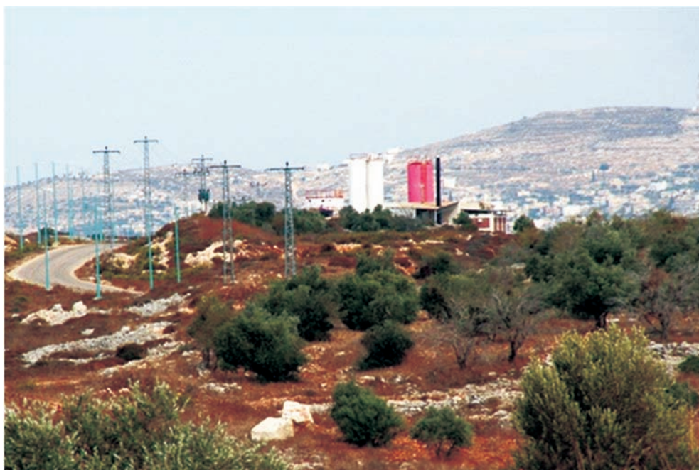
Figure 15: Off-site perspectives for chemical disaster risk and vulnerability.
