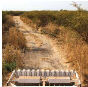
PICTURE A1.1 Road clearance; South Sudan. UN Photo
