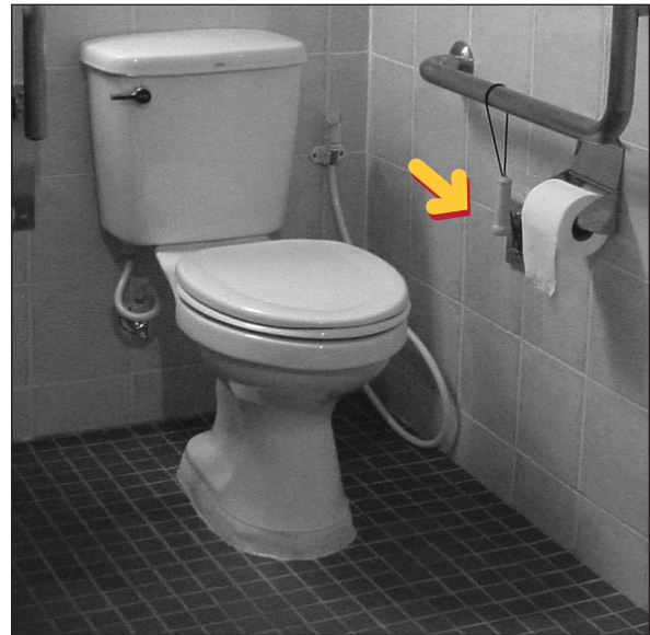
Fig. 35: Emergency system for restrooms / toilets
