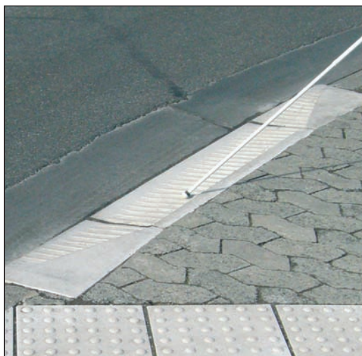
Fig. 39: High contrasting, tactile and bevelled applications on pedestrian way
